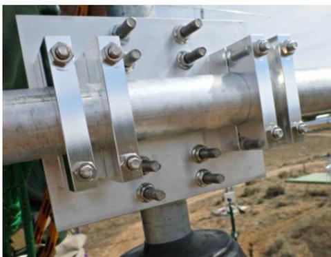
*Boom to Mast Plate attached to Boom
