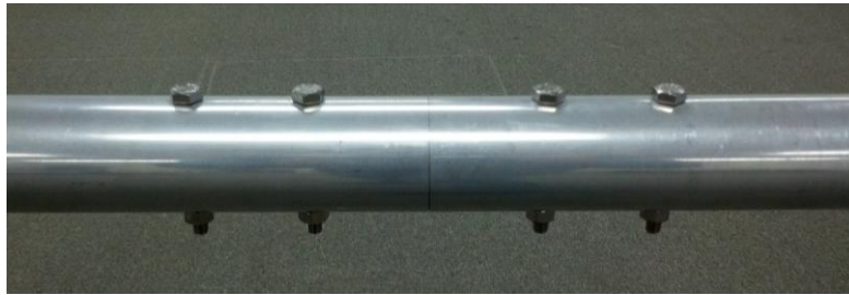
Assembled Boom Joint
